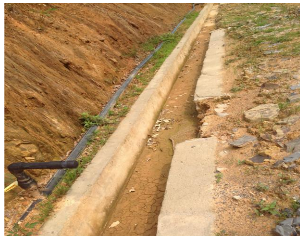
场区西面撇洪沟
